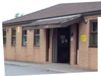
Patchway Health Centre
